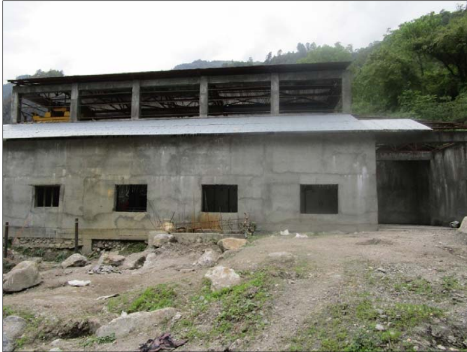
Pic-19 Side view of Power House
