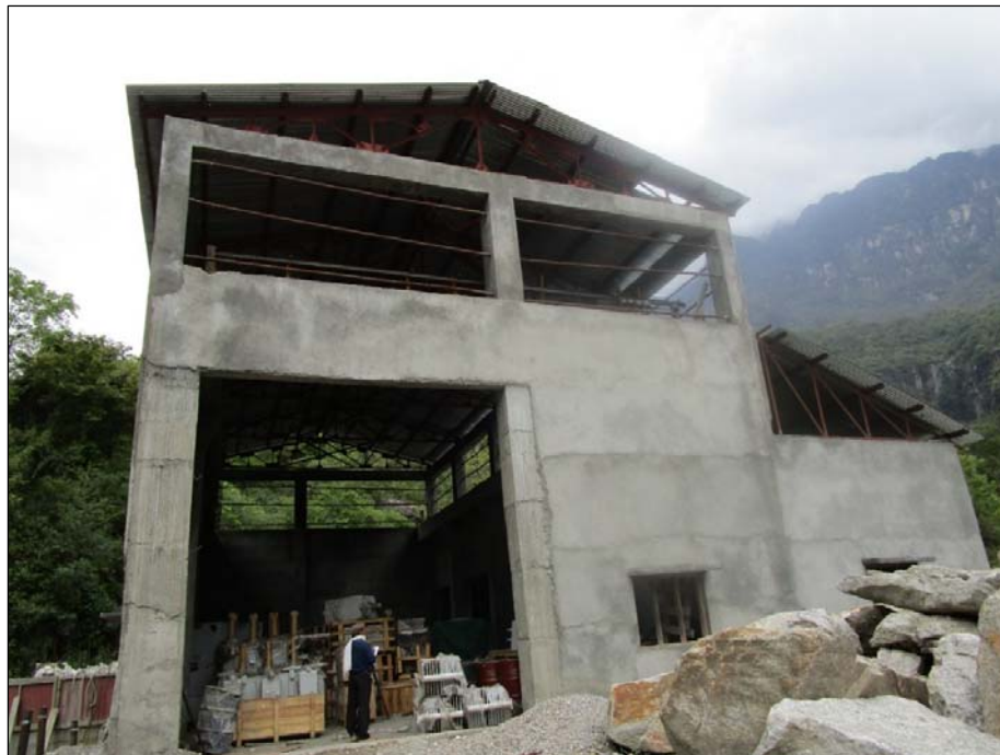
Pic-18 Outer view of Power House
