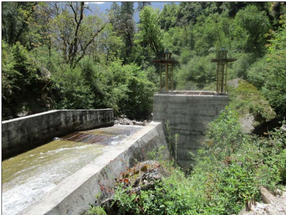
Pic-2: Trench weir
