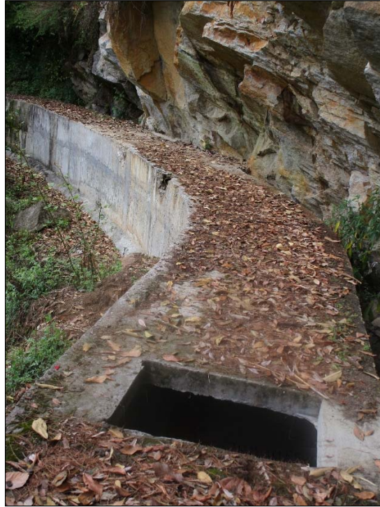
Pic-7 Opening for Inspection on Power Channel
