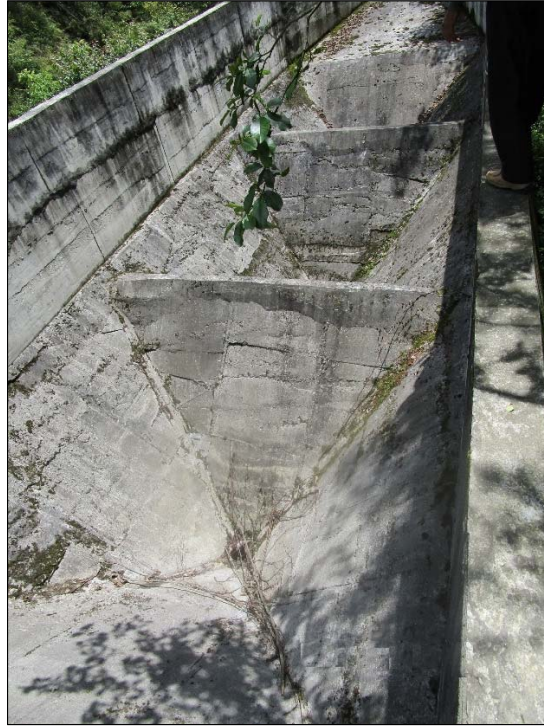
Pic-5 Desilting Tank
