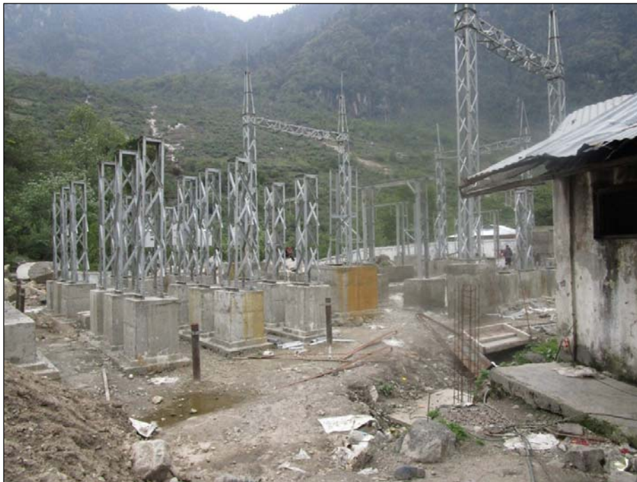
Pic-26 View of Switchyard (under construction)
