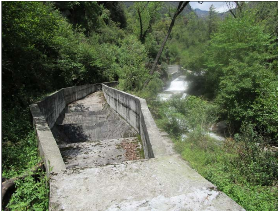
Pic-6 Another view of Desilting Tank
