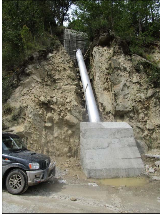
Pic-15 Anchor Block at Penstock
