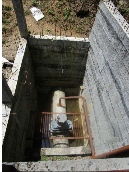
Pic-13 Control Valve at head of Penstock
