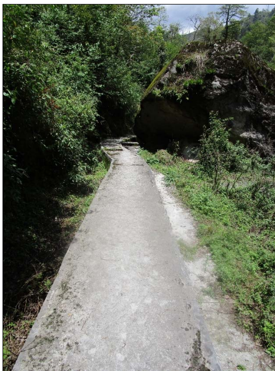
Pic-4 Feeder Channel
