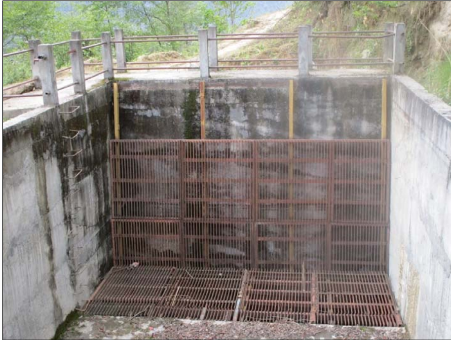
Pic-11 Another view of Forebay
