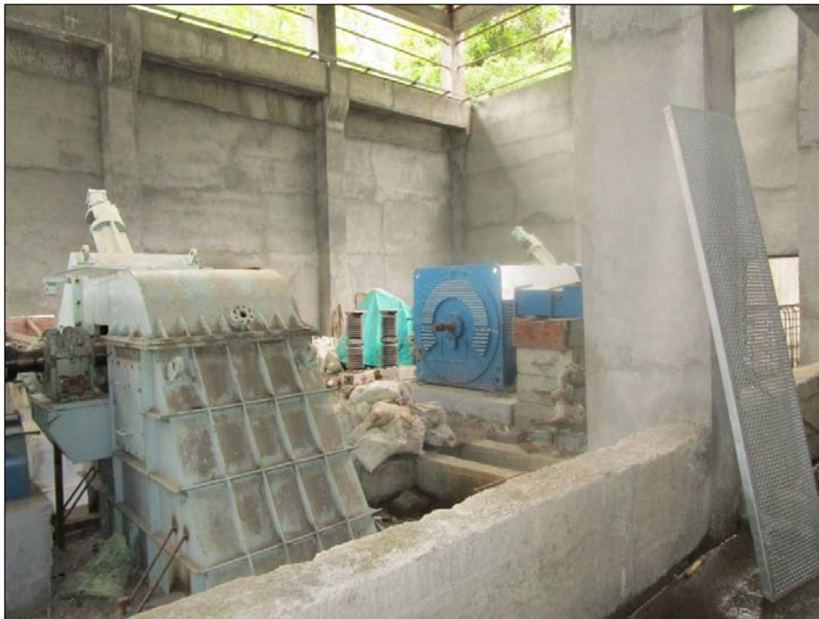
Pic-20 Inside view of Power House
