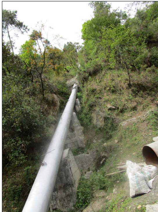
Pic-16 Supports below Penstock
